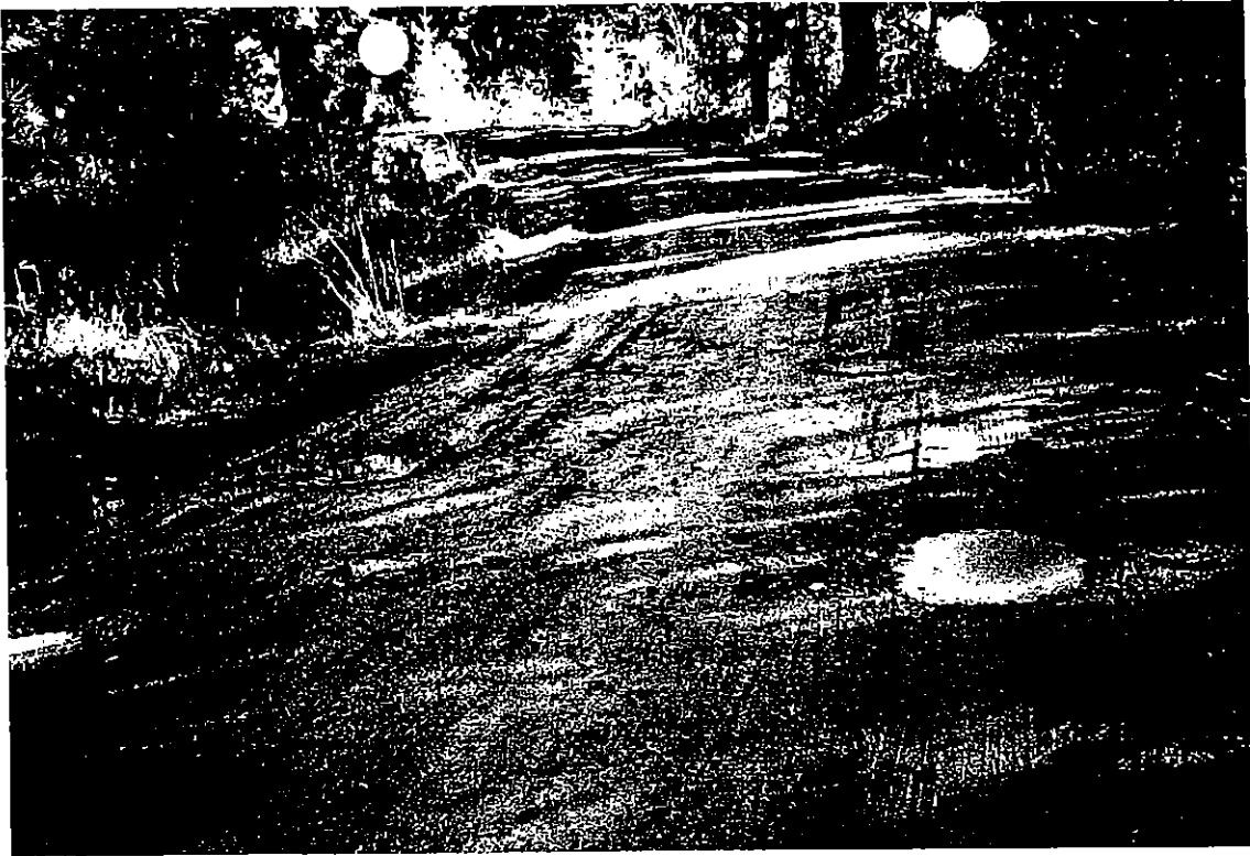
Cedarcroft Road-note poor condition
