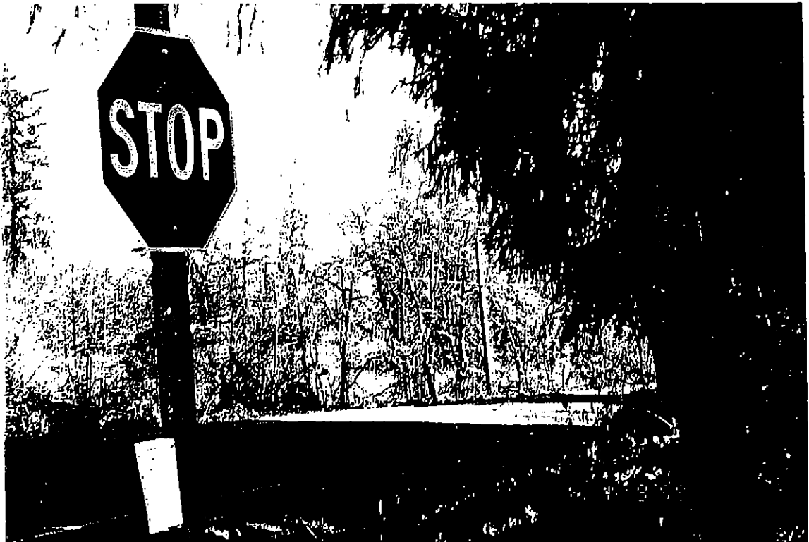
Intersection of Bradford Rd. and Bear Creek Rd looking east: Note how shade makes visibility even more difficult
